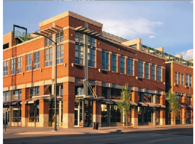
103. Retail and facade ornamentation on the Lower Story Facade of the building mask a parking structure, effectively screening views of parked cars and providing an active street environment for the pedestrian.
